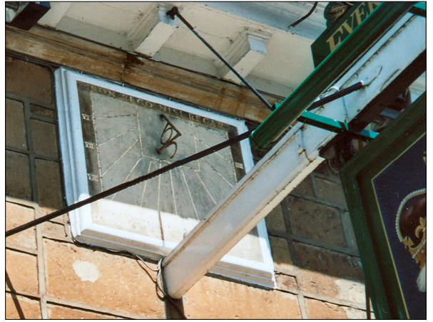
Fig. 5. The dial on the Crown Hotel, High St East, Uppingham. Dated to the early 19 th century, it is now badly overshadowed and has a broken gnomon. Its motto 'Non Rego Nisi Regar' translates to 'I do not guide unless I am guided'.
