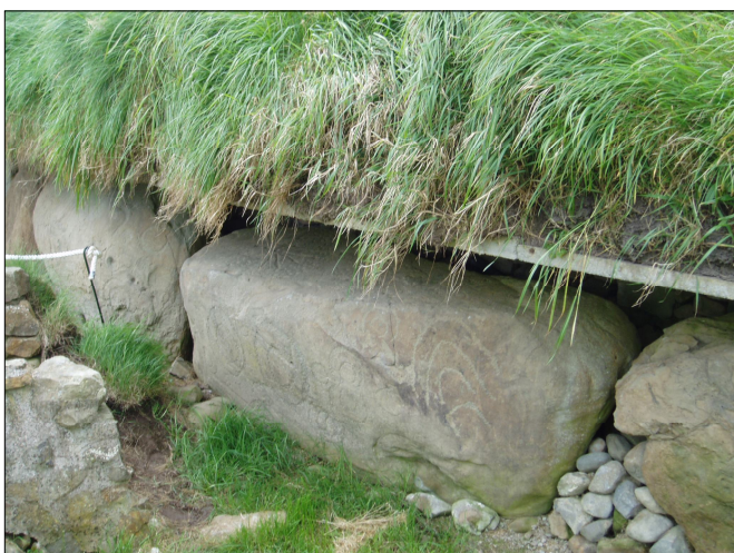
Fig. 11. Projecting concrete ledge over Kerbstone K7.
